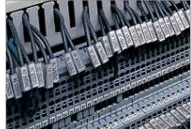
Easy configuration and testing using 1-pole female plugs.
