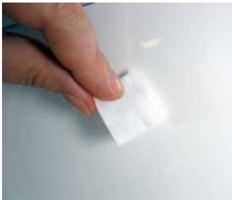
Figure 17. Adhesive Mount Antenna – Step 1. Pre-clean the surface
